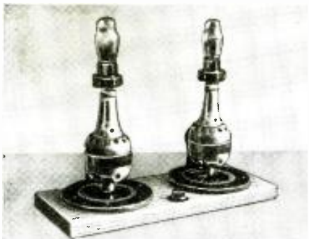
These vibrators give tubes as much shaking in a few minutes as they receive in thousands of miles of use in auto radio sets. Any rattles or poor welds soon show up.
